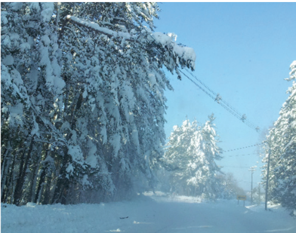
Ice and snow loading on a tree overhead corridor.
