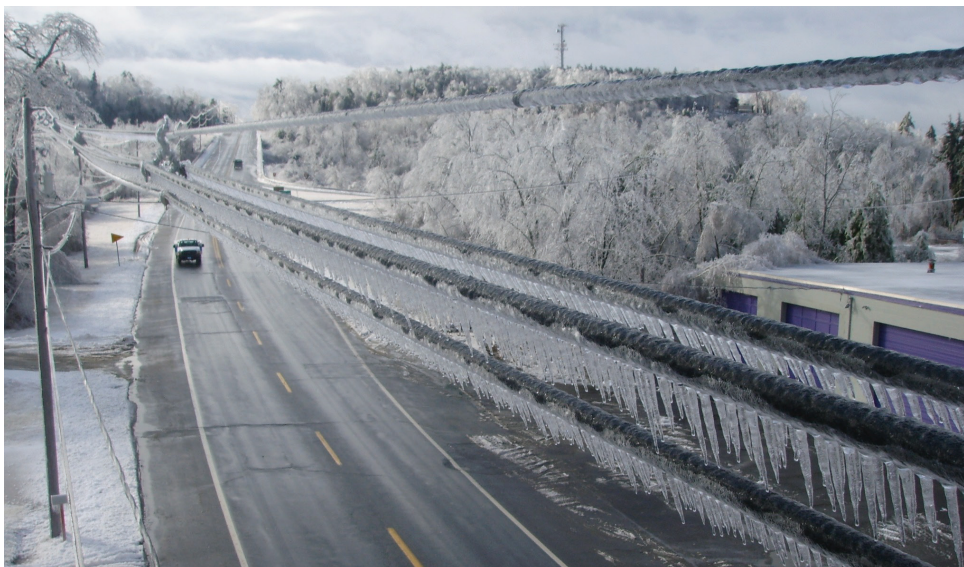
Ice accumulation along a Templeton, Massachusetts corridor during the December 2008 event.
