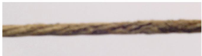
Photo 2: Galvanized Messenger in Dry Pacific Seacoast Environment after Only 9 Months
