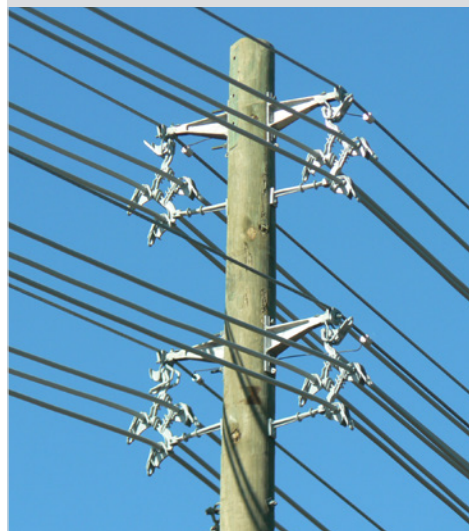
Multiple circuits reduce clearance requirements
