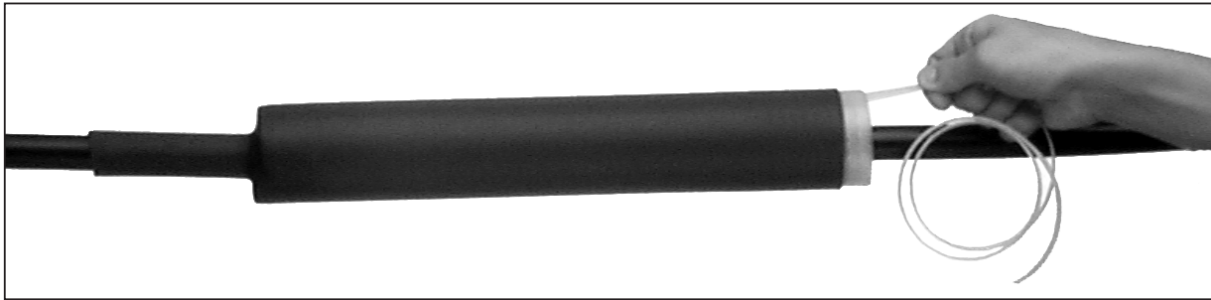
Removing the core
