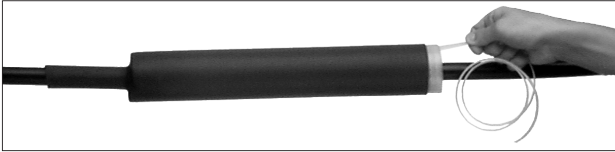
Removing the core
