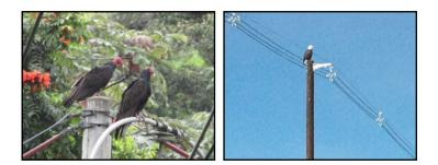
There are cases where a flock of birds sitting on a powerline alight simultaneously and cause a flashover between phases. This is not possible with covered conductor systems, due to the protection afforded by the insulation.
