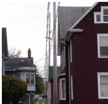
Clearance Issues & Limited Right-of-Way
